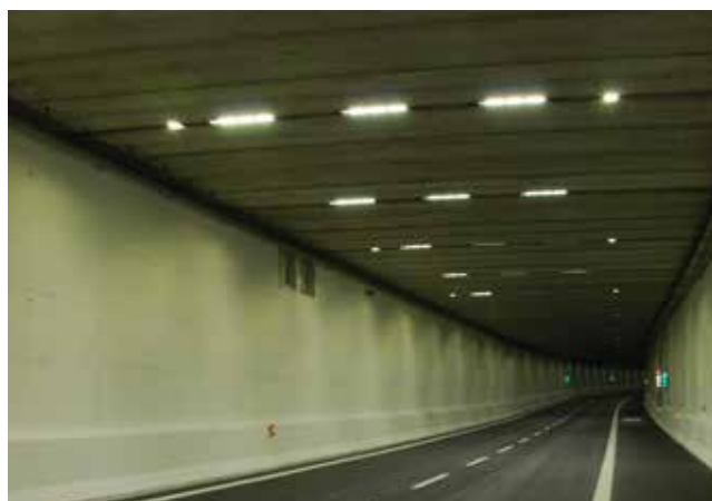
EXPO 2015 - MERLATA TUNNEL
